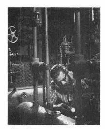
OIL LEVEL in compressor is checked several times during the 4 p.m.-midnight maintenance shift by Henry Flowers (4511-2). He checks and maintains operation of environmental test chamber in Area II.
